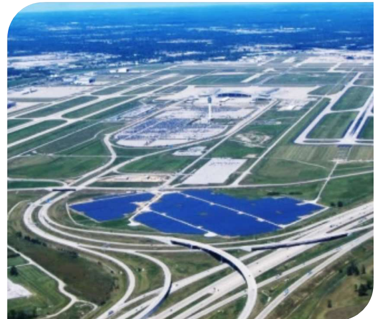
25MW Cenergy installation at Indianapolis Airport
